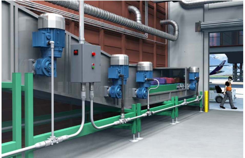
In this application a, a high-power line feeds cables that take it up to individual blue-colored drives.
