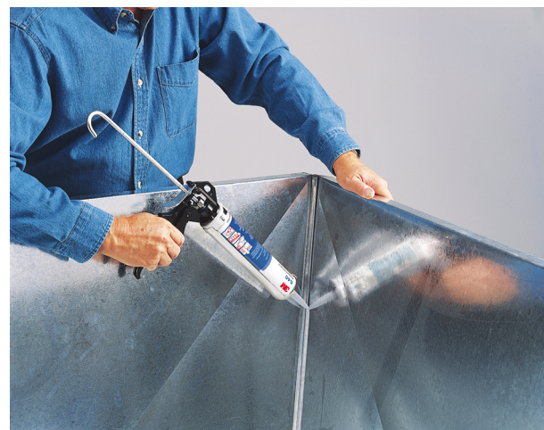
Adhesive sealants can fill voids left by mechanical fasteners.
