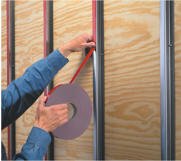
Adhesives and tapes provide the holding strength, flexibility, and gap-filling necessary for panel-to-frame assemblies.
